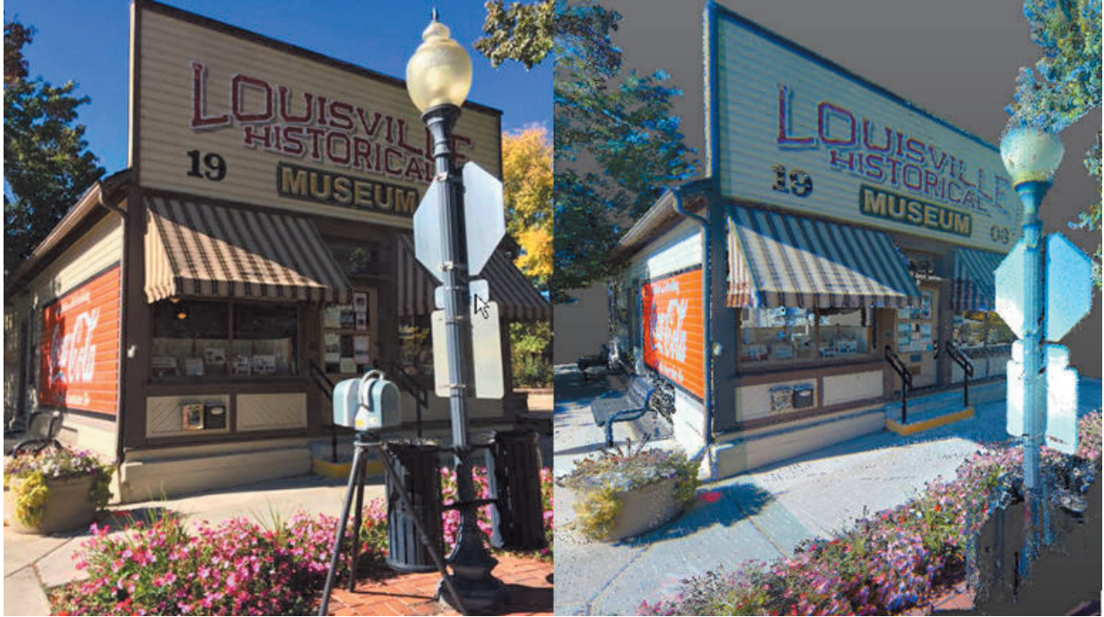
Figure 3: TX6 colored point cloud of building exterior.
