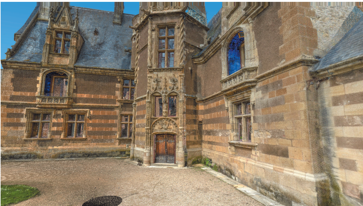
Figure 2: TX8 colored point cloud of a 14th century castle, Chateau d'Ainay-le-Vieil
